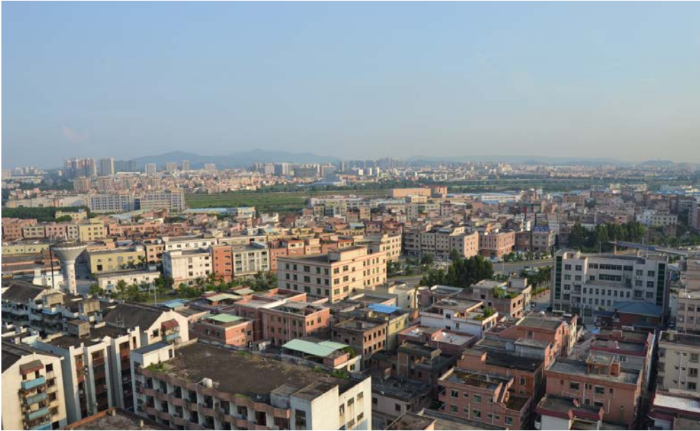
FIGURE 4: Jian Sha Zhou's emerging urban fabric. Image credit: Timo Heinonen and Tian Xuezhong
